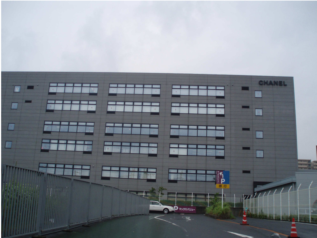
Photo 2 Chanel Corporate Operations Center, Funabashi: A building complex housing three functions, including a cosmetics technology development Institute, a training center, and a distribution center (photo taken by the author in July, 2008)
